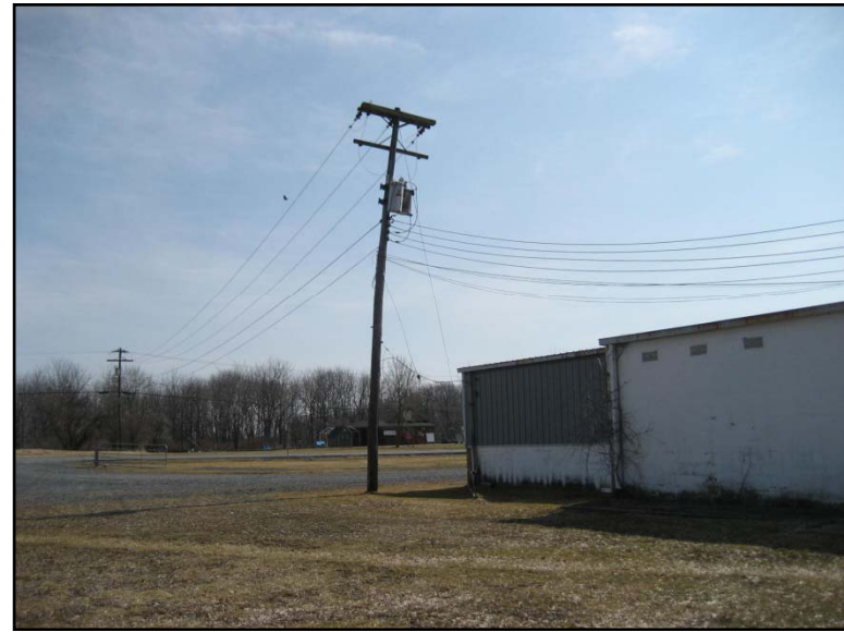
Photograph 4: Pole-type transformer on subject property.
