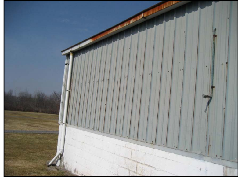
Photograph 2: Boat repair shop exterior showing roof leader drain.
