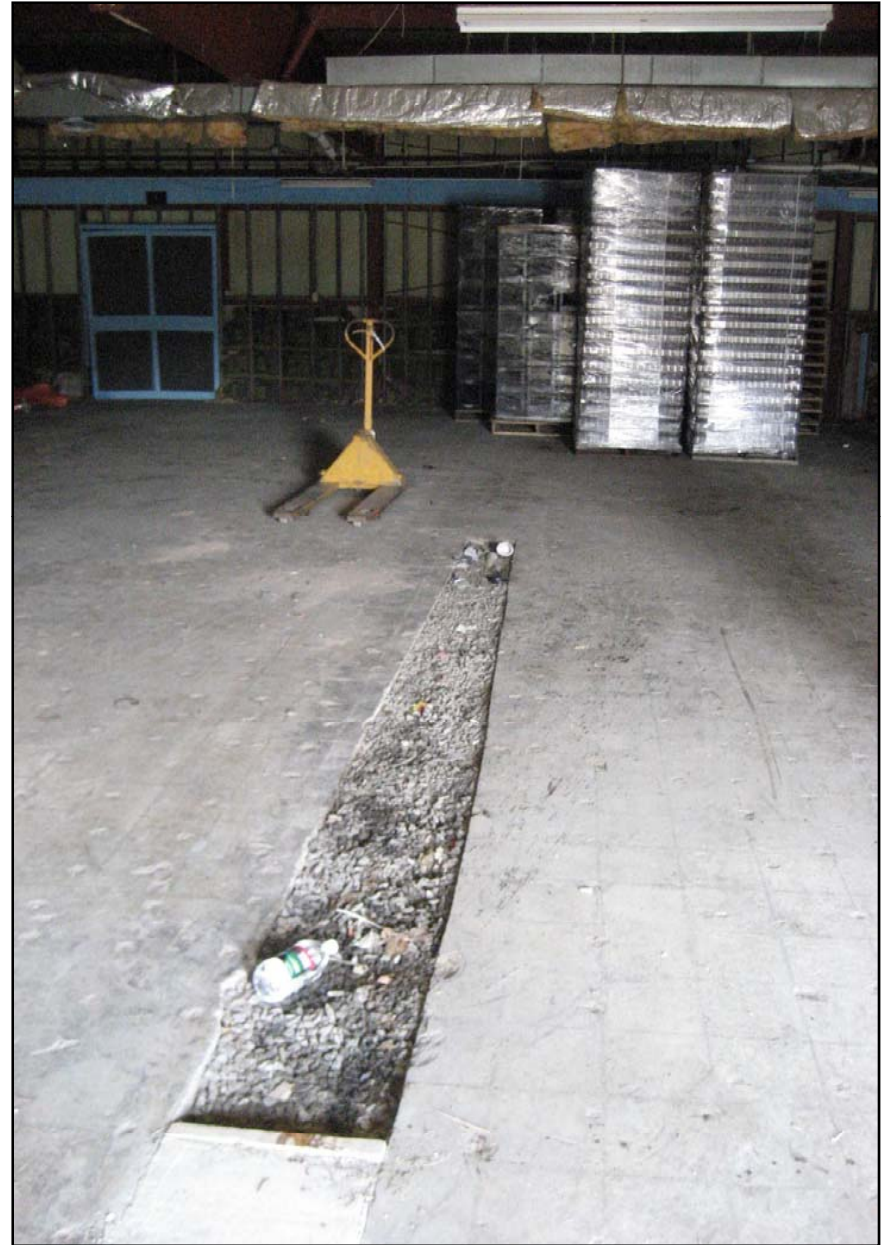
Photograph 7: Interior of the boat repair shop, including thermal system insulation, tile flooring and trench drain.
